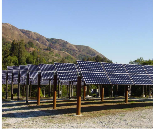
Figure 1: Single Axis tracking system. Photo Courtesy RayTracker
